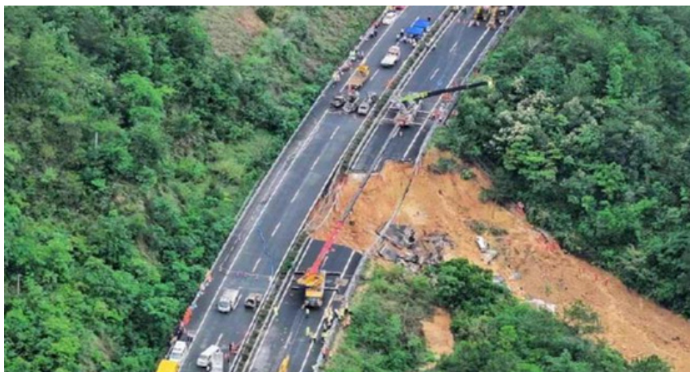
Figure 5. At around 2 o'clock on May 1, 2024, the Chayang section of Meida Expressway in Meizhou City, Guangdong, China, collapsed. By 14:00 on 2 May, 23 vehicles had been found down and 48 people had died.
